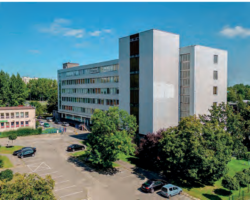
Budynek D – widok od strony parkingu wewnętrzny / Building D – a view from the internal car park, fot./photo A. Wisniewski
